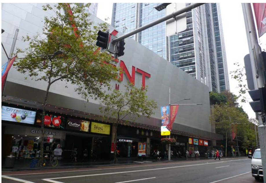
Figure 3 – George Street Elevation of the existing Building
