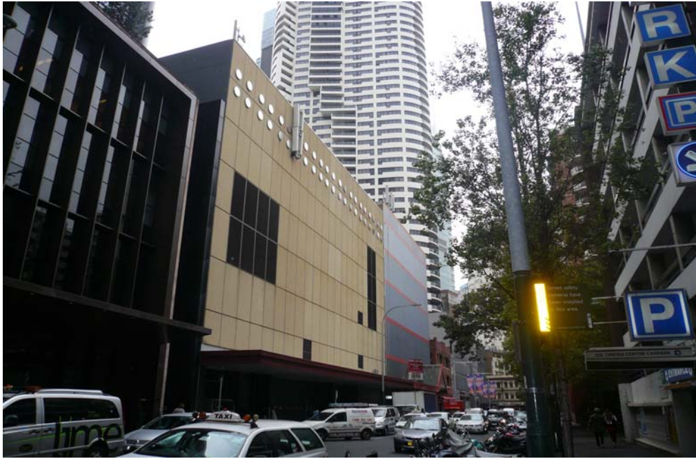
Figure 4 – Kent Street Elevation of the Existing Building
